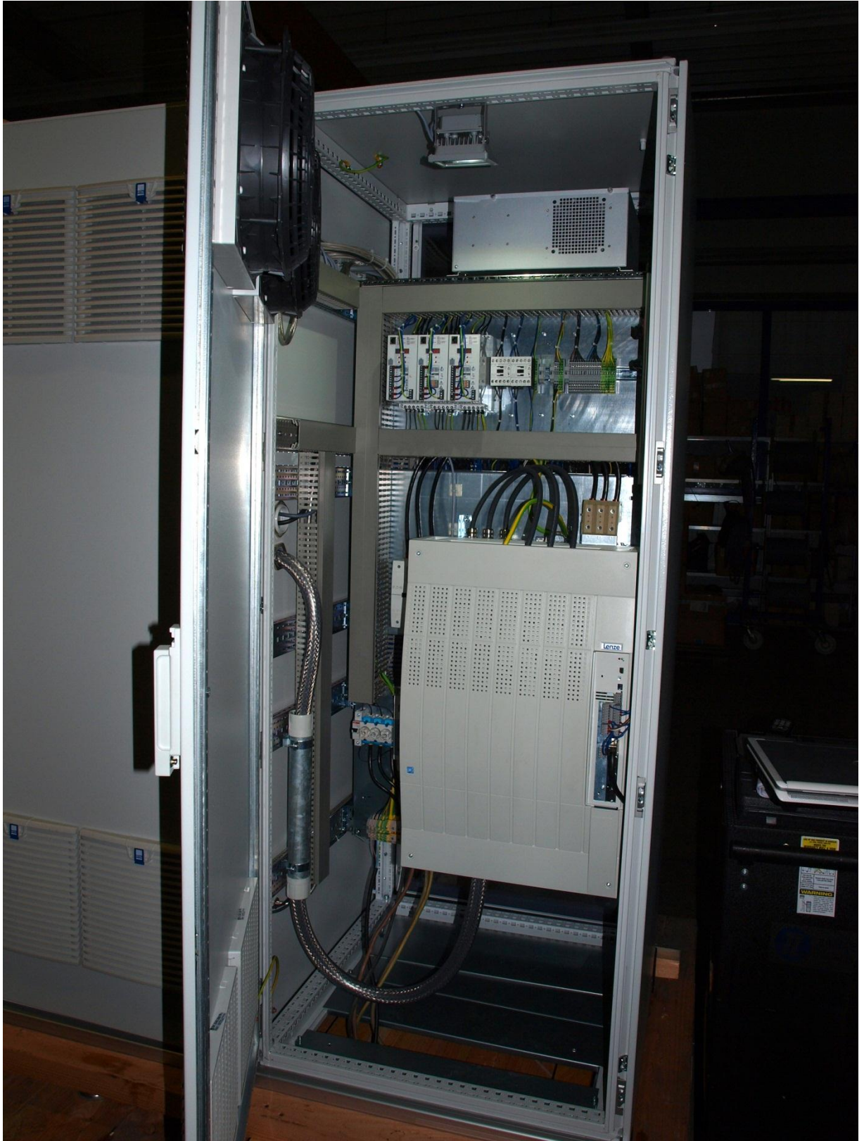
Figure 7. Module of the power electronics
